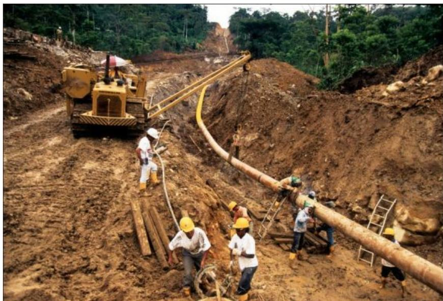
Construction of an oil pipeline in the Ecuadorian Amazon by Arco-Oriente that carries 80,000 barrels of crude oil from the Villano oil reserve to the TransEcuadorian pipeline. Pipeline ruptures in Ecuador have discharged over 18 million gallons of oil--more than the 10.8 million gallon Exxon Valdez spill. Photo (c) Bruce Farnsworth.
